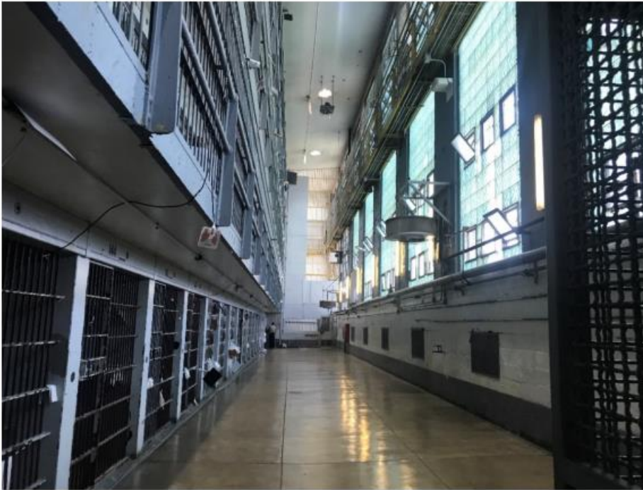
PHOTO # 1 & 2 – View of Catwalk Level Enclosure & Gallery from Ground Floor
